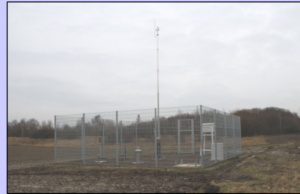
Abb. 1: Neue Klimastation RGS-2
